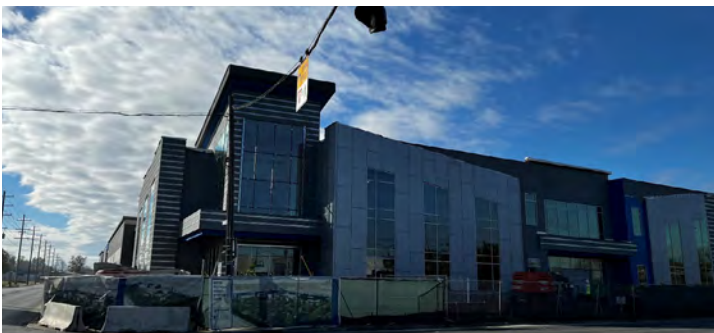
Exterior construction is still ongoing.
