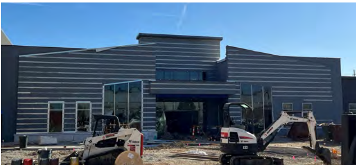
Development of outdoor plaza is ongoing.
